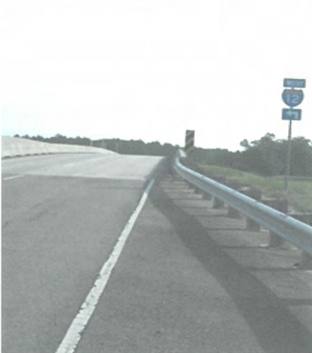
Figure 4: Overpass Shoulder Disappears
