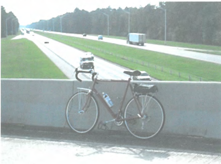
Figure 6: 1088 I-12 Overpass Retaining Wall
