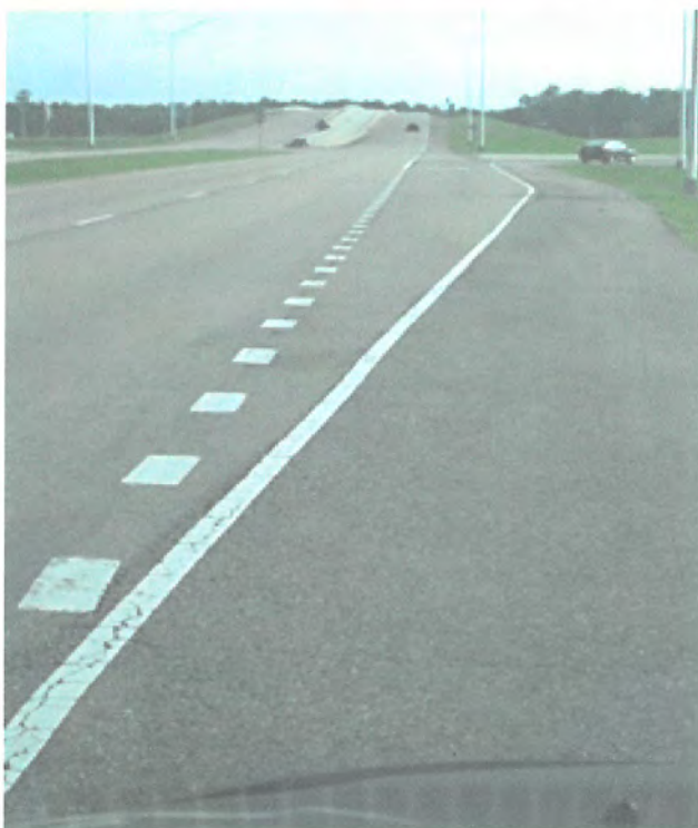
Figure 3: Approaching the I-12 eastbound on-ramp
