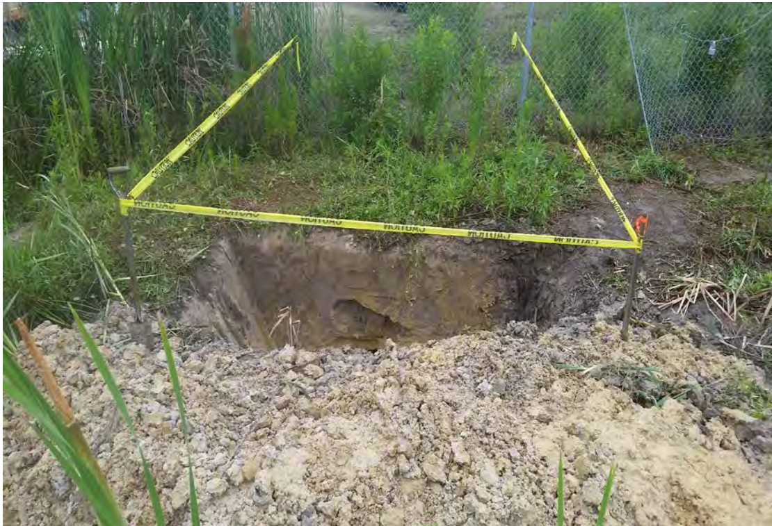
Photo 3: Utility work and soils found near intersection of I-12 and LA-1088. Photo was taken looking west.
