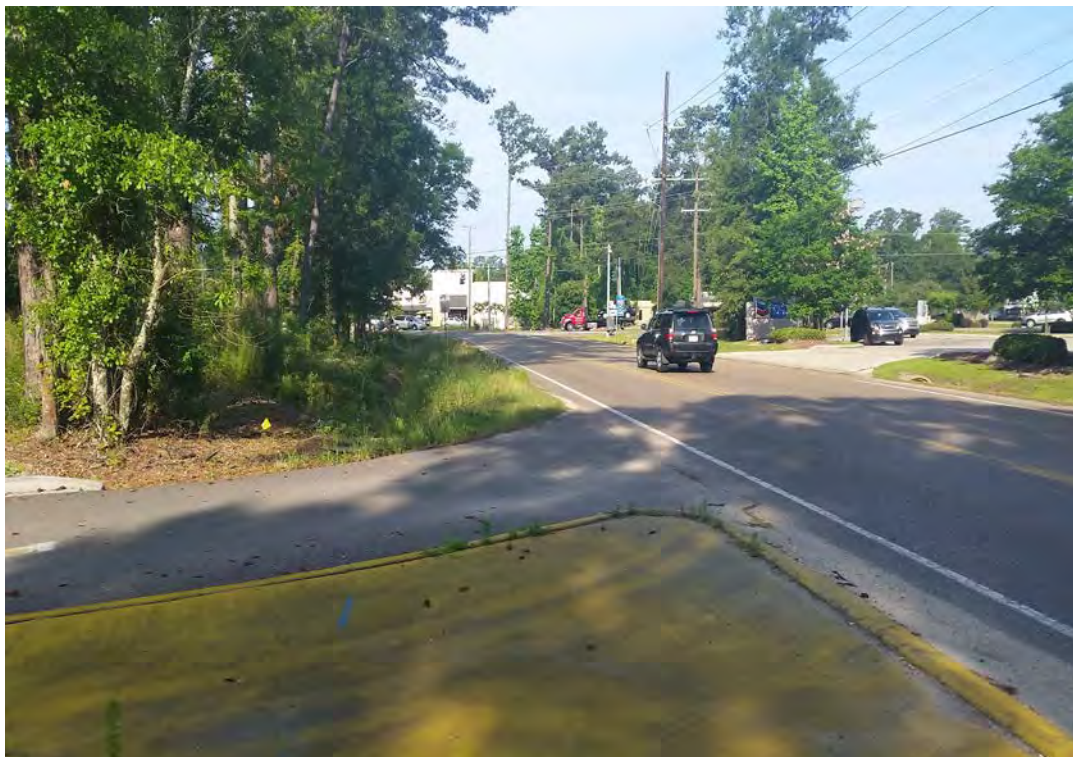
Photo 40: View along LA-1088 looking south towards the intersection of LA-59.
