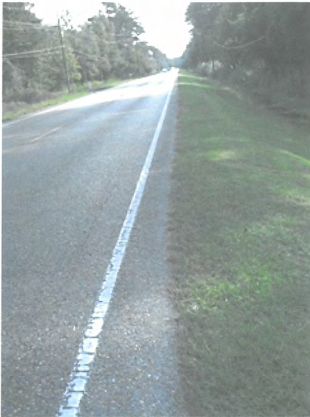
Figure 1: 1088 Roadway at Quail Creek
